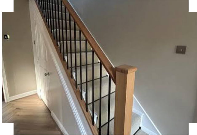
OAK DOORS, HANDRAIL, BASERAIL & NEWAL POST TO STAIRCASE
