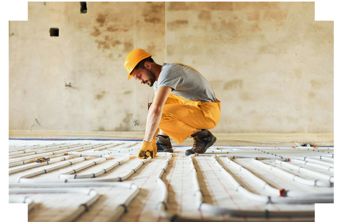
UNDERFLOOR HEATING TO THE GROUND FLOOR
